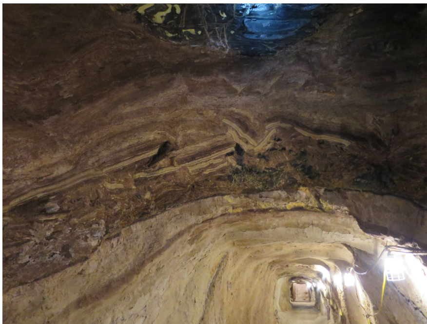
Mine-collapse horizon. After coal seams were mined out and the pillar pulled, the mines sometimes collapsed. Later, when they cut new tunnel for sand mining, they intersected some of the old collapsed coal adits.
